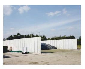
also has the ability to act as a retaining structure in applications such as ground walling, perimeter boundaries and changes in levels. Rockwall retaining units can be cast in to new concrete slabs or anchored down to new or existing concrete foundations.
