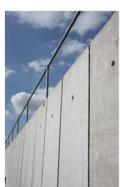
station. Rockwall also has the basic ability to act as a retaining structure in general applications such as ground walling, perimeter boundaries and changes in levels, mainly where constraints such as access and time are paramount. The Rockwall retaining units can be cast in to new concrete slabs or anchored down to new or existing concrete foundations.
