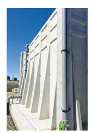
arrangements. The units have a unique jointing system that ensures a watertight and secure connection between adjacent panels. Meeting the stringent requirements of both BS 8007 and EC2, our Sealwall units are largely used within the water industry as sludge, storm overflow and sewage tanks.
